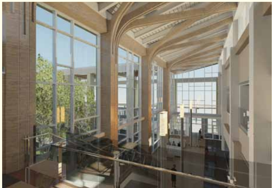
Upper atrium of Colchester Regional Hospital in Truro, Nova Scotia (photo courtesy Farrow Partnership)
